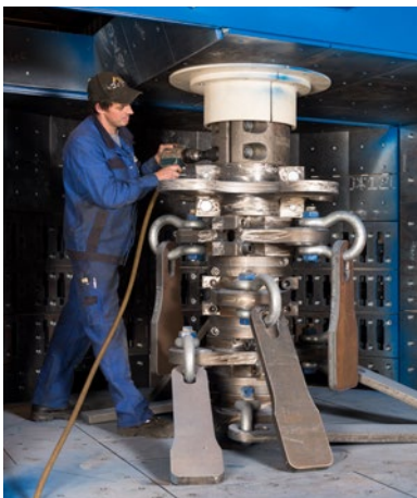
Specialized personnel during installation
