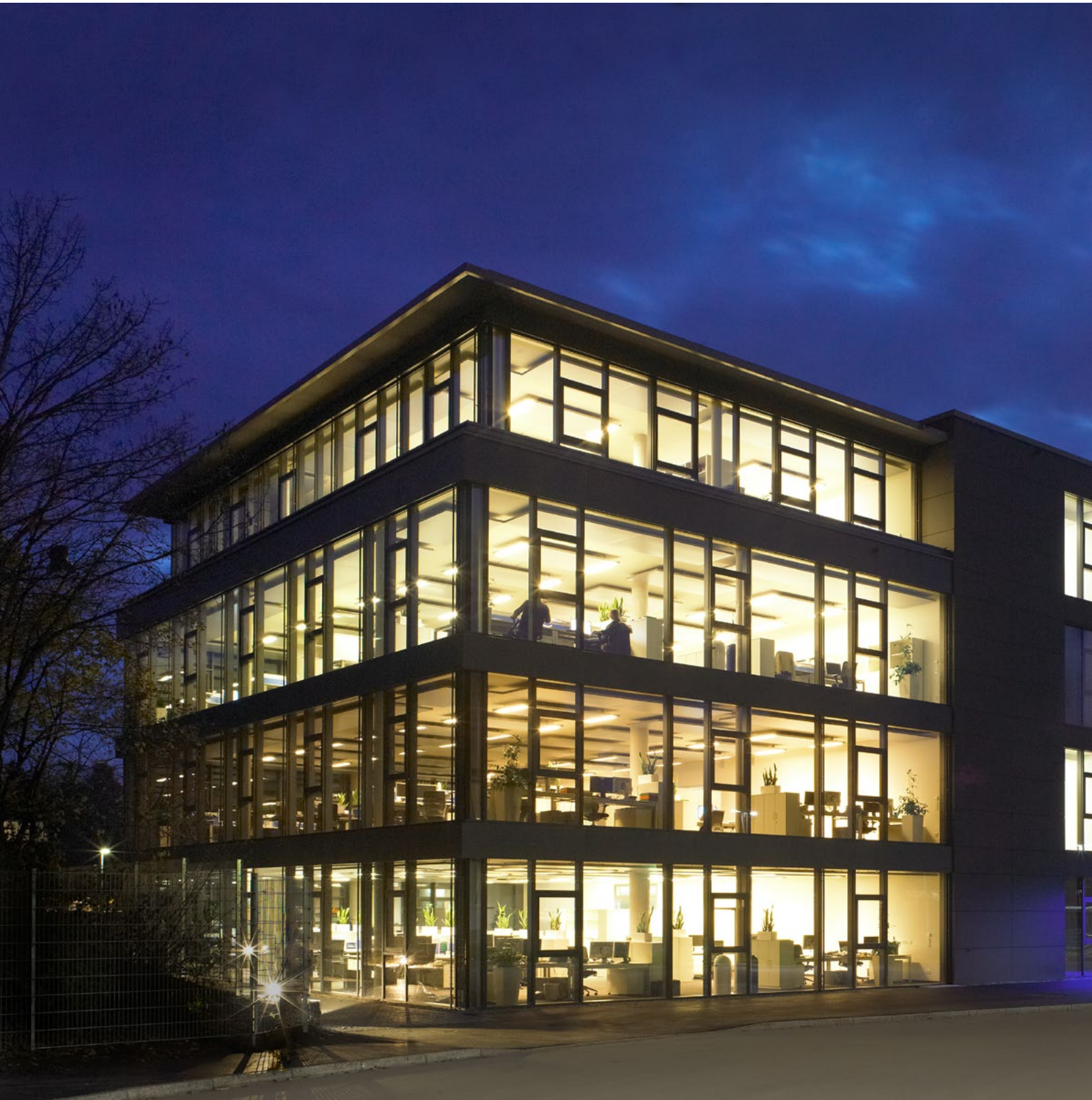
Headquarter of BHS-Sonthofen in Germany
